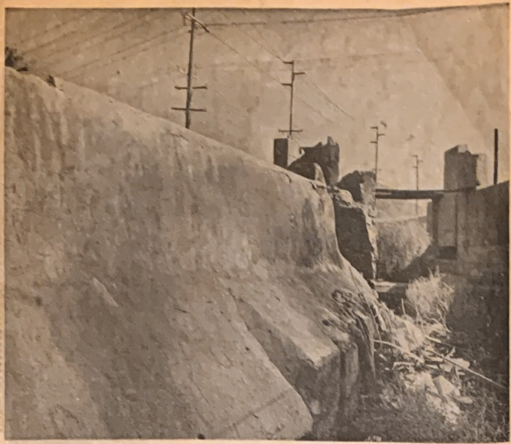
TODAY — Left picture shows the overflow of the Highgrove water plant today. Water doesn't overflow, however, because it passes
