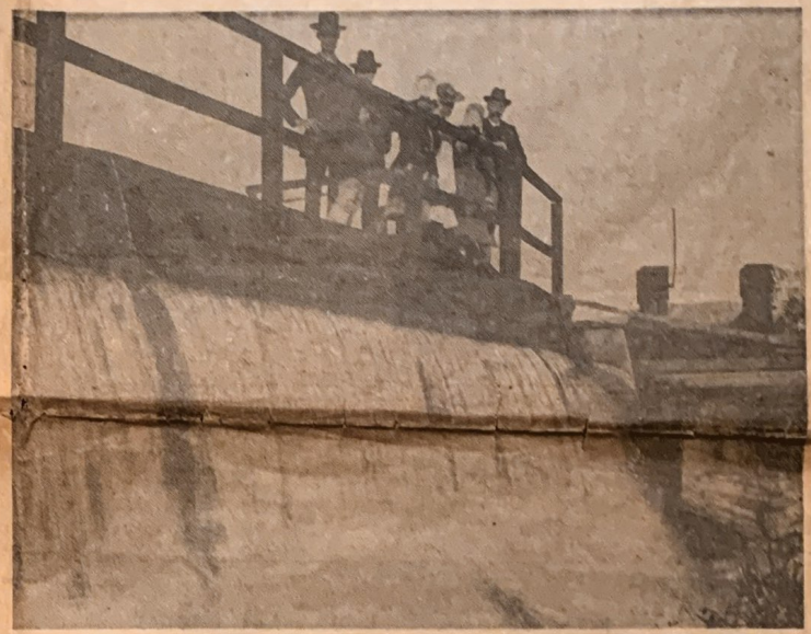
OVERFLOW — This was the overflow at the forebay, where the canal enters the penstock. The bypass channel is on the right. Edith McCright and her father, Charles F. McCright, a citrus grower, are among the people in the picture.
